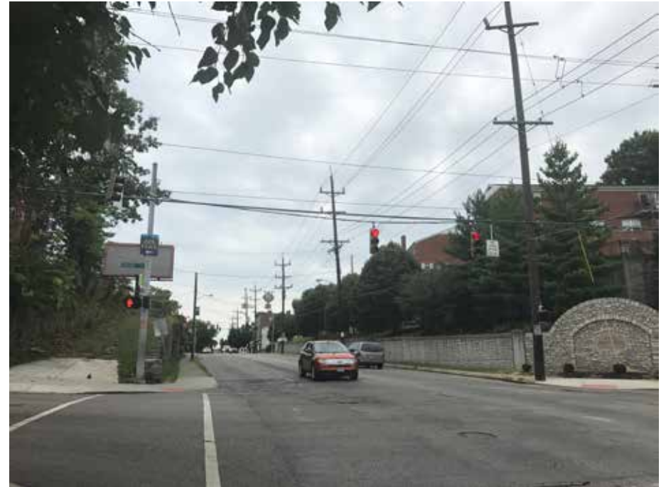
Existing conditions at the intersection of Warsaw Avenue and Grand Avenue
